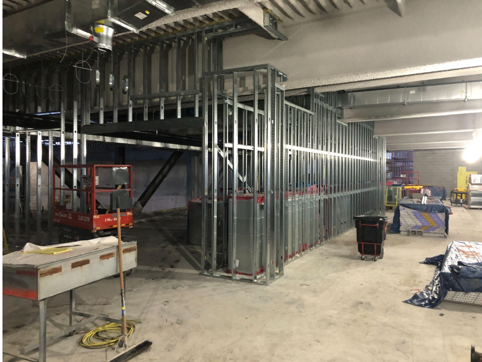
Interior Framing of Cardio Classroom
